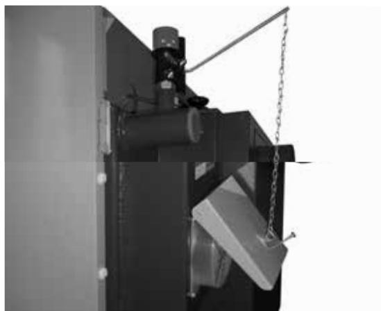
View on air duct with air control flap and draught regulator FR124
