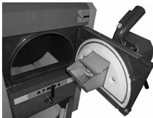
Open top door of the boiler during cleaning of the combustion chamber of the burner
