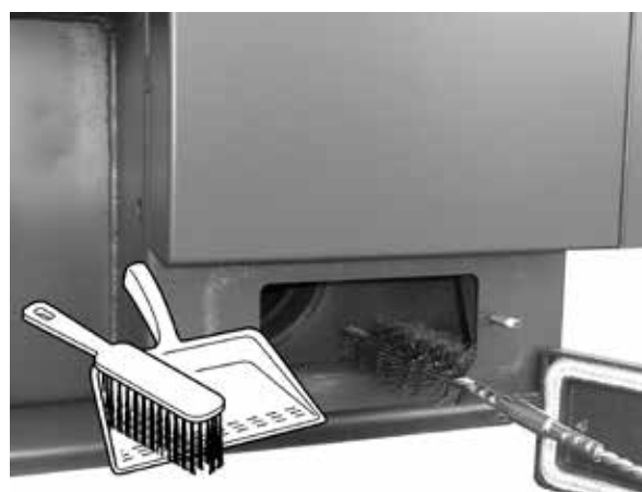
Open bottom cleaning lid on the smoke channel
